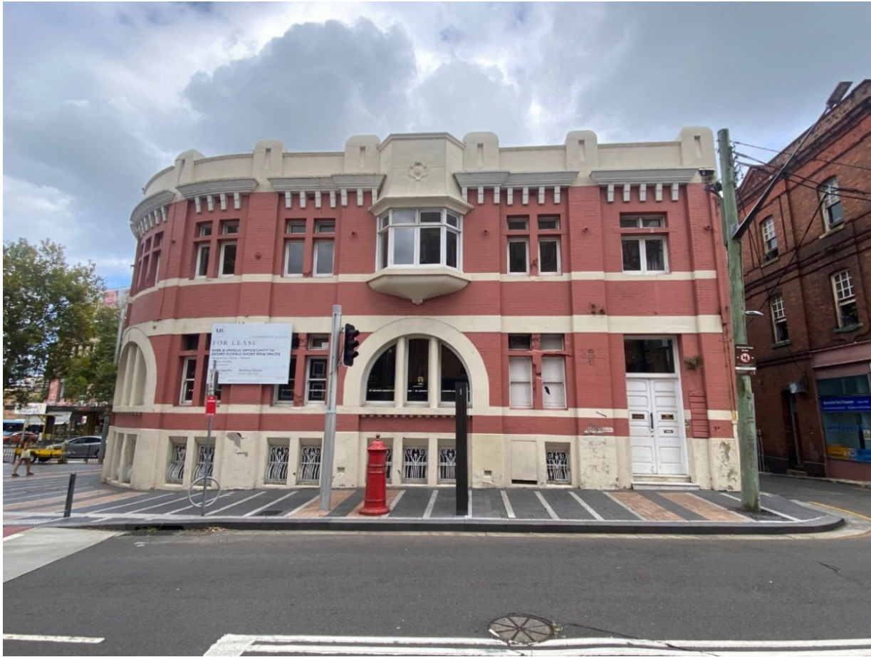
site viewed from Bourke Street
