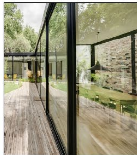
D - ALUMINIUM FRAMED GLAZING
